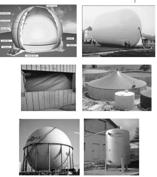
**Figure 2.1** Gasholders. Double membrane gasholder (pat.)<sup>3)</sup> (top left); Bag bio gasholder (top right) Enclosed theomoplastic foil gasholder (middle left); Theomoplastic foil gasholder on a bioreactor (middle right) Cube gasholder (below left); Steel tank gasholder (below right)
