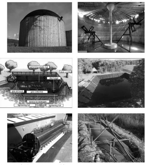
Figure 1.1 Reinforced concrete in Europe (top left), Heating and agitation devices inside a vertical bioreactor (top right), Construction of a basin (middle left), Uncovered basin (middle right),
