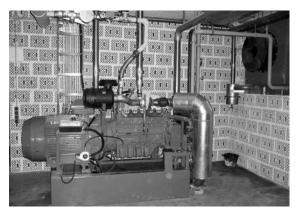
Figure 1.4 Sound-absorbing wall.
