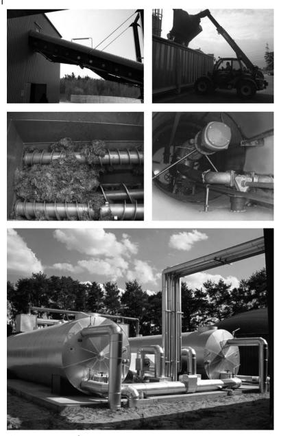
Figure 3.8 Equipment for upstream processing Closed belt conveyor (above left), Feeding the bioreactor (above right) Feeder (vielfra $\beta^{\otimes}$ ) for agricultural plant (middle left), Pump chute (middle right), Hygienization installation (below).
