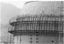
**Figure 4.24** Digestion towers. Bioreactors for the degradation of sewage sludge-*Classical form (top), modern form (middle), Climbing formwork-Digestion tank in Munich (Germany)-Digestion tank in Pa-Li (Taiwan).*
